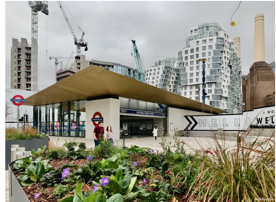
Battersea Power Station underground extension – privately financed
